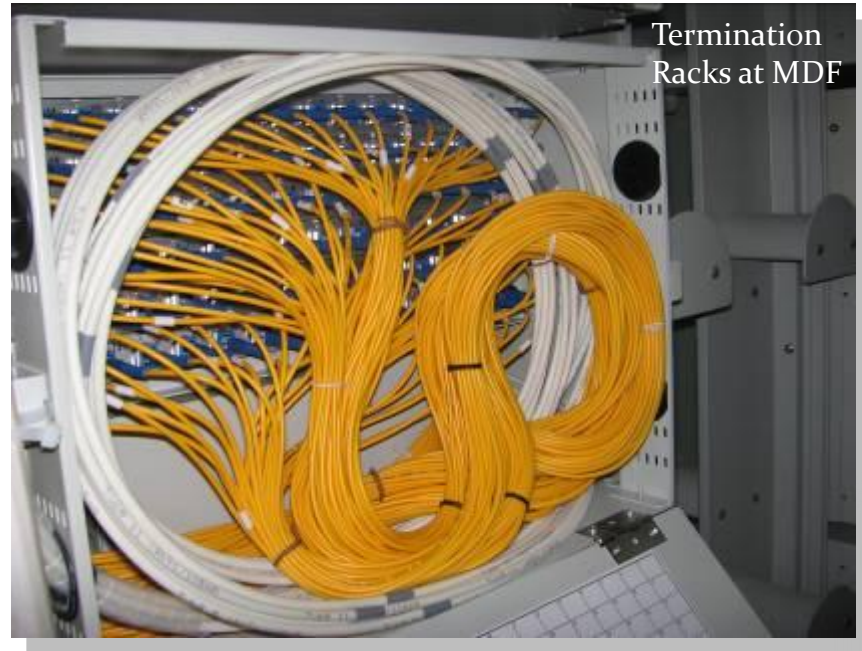
Termination Racks at MDF (~1000 units)
